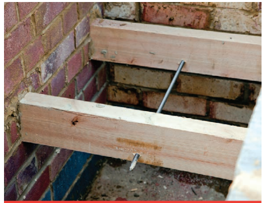
BowTie HDs installed through parallel floor joists
