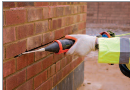
5. Inject into the slot or hole in a continuous operation. Typical working life of the mixture in the pail is around 2 hours with re-agitation . The cartridge should be emptied within 5 minutes. If the injection process is interrupted for any reason, empty any cartridge contents back into the bucket and re-mix until it again reaches a smooth injectable consistency
