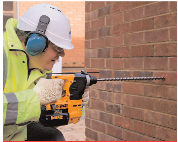
Drilling clearance hole in both wythes ready for CemenTie installation
